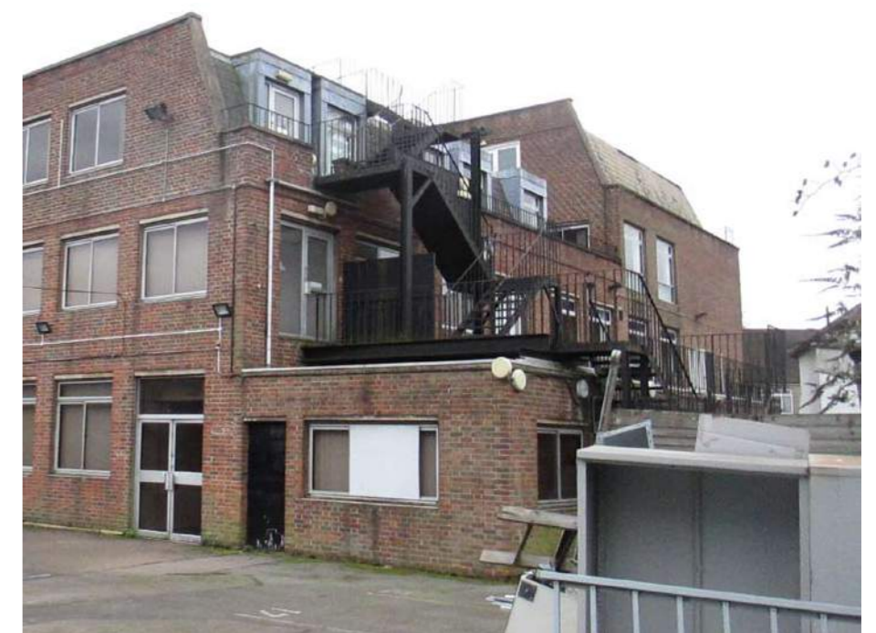
Existing external escape stair on side elevation (North West)
