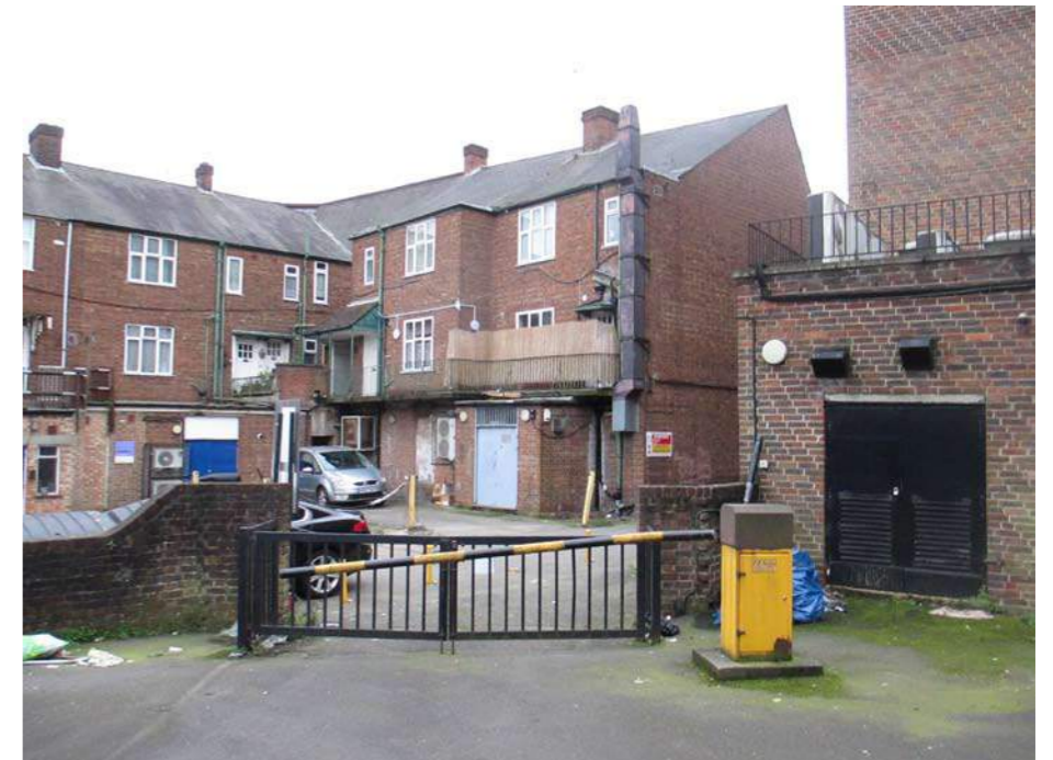
Existing access into car park via barrier arm and gate
