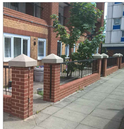
Example of Garden Wall to be Replicated
