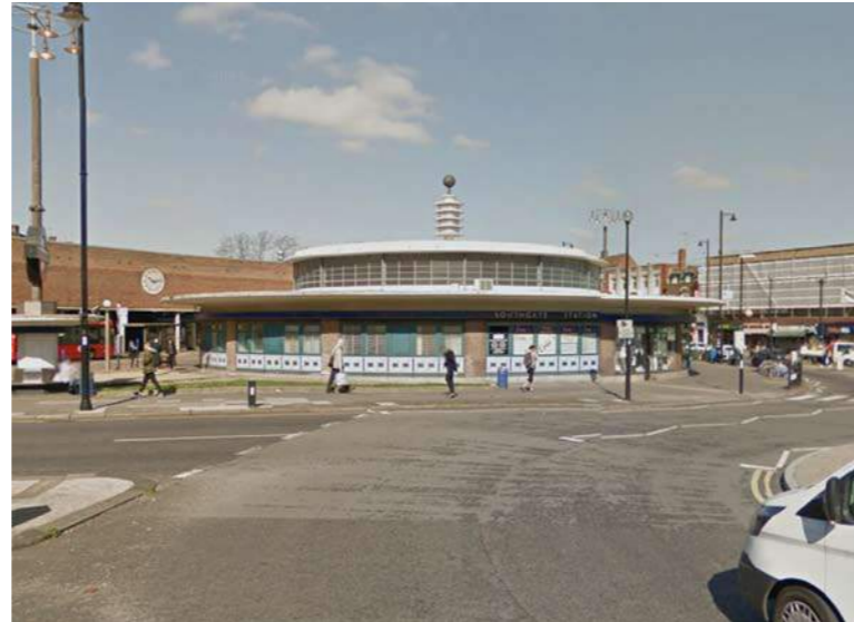
1. Southgate Underground Station from East
