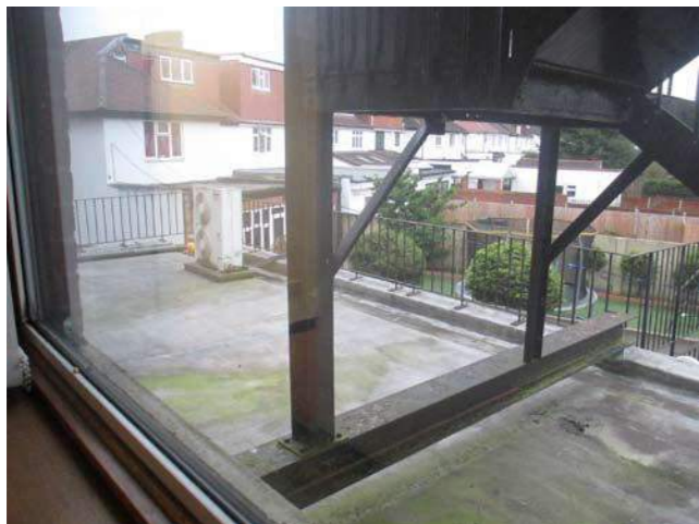
Existing view of no. 91 from first storey
