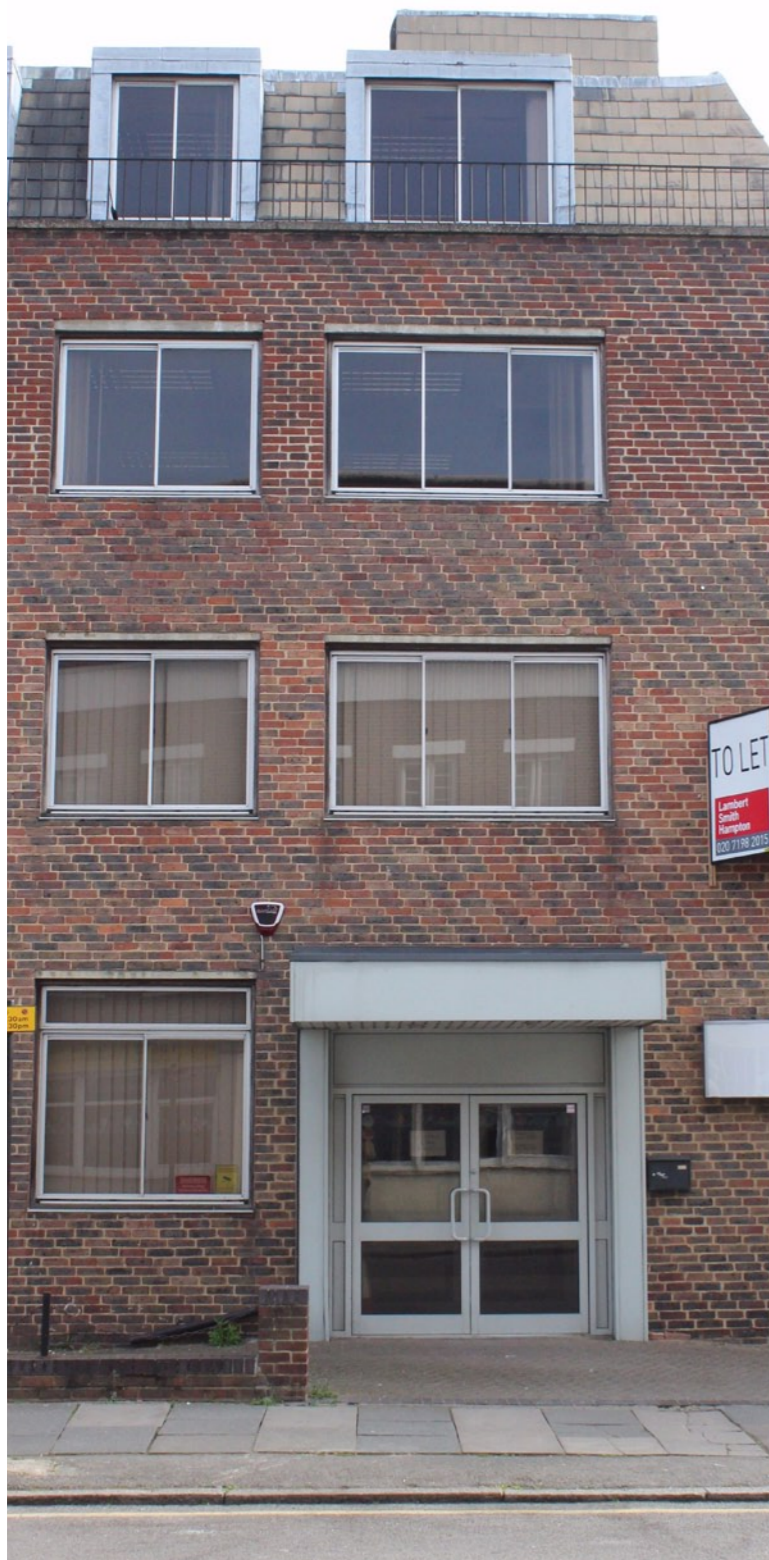
Existing entrance canopy
