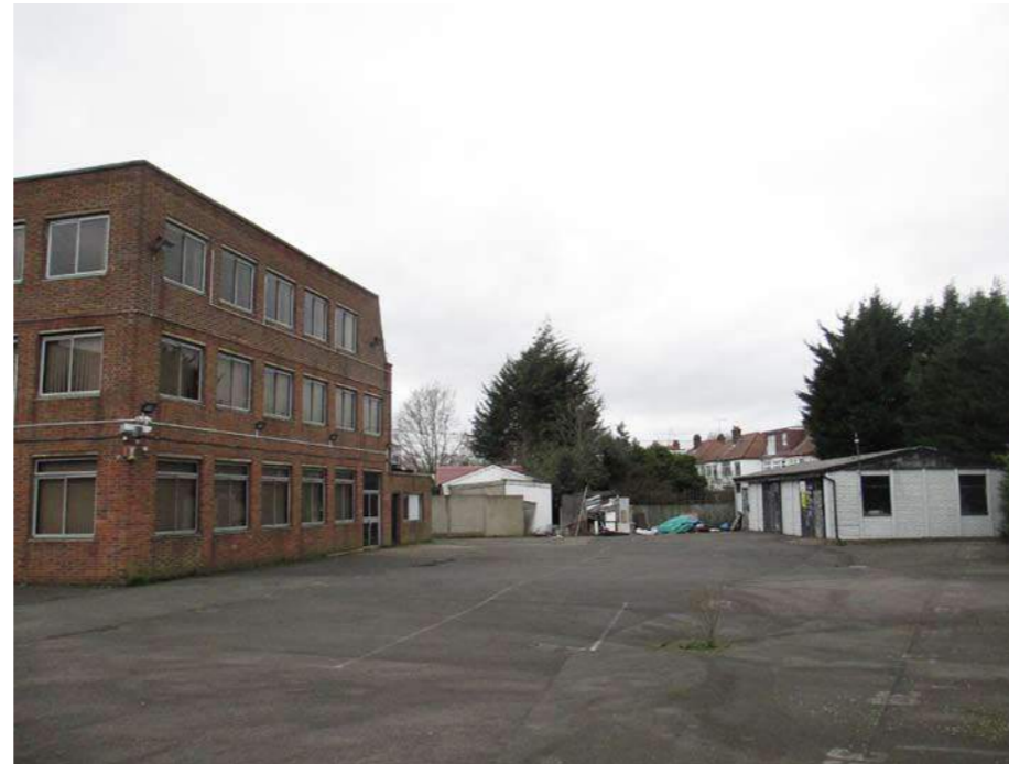
View across existing car parking to outbuilding at rear
