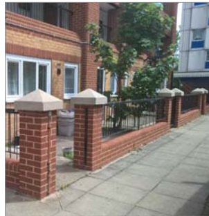
Example of Garden Wall to be Replicated
