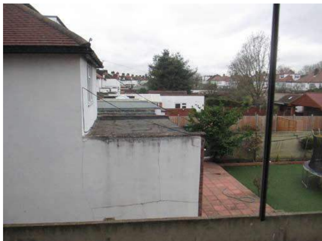
Existing view of no. 91 from first storey
