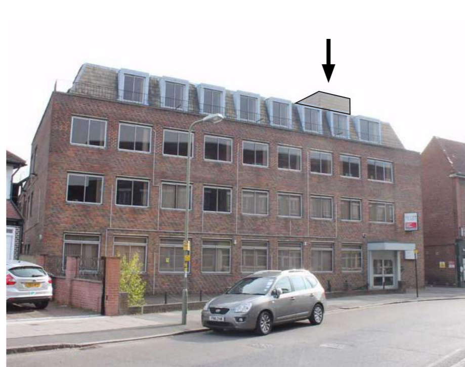
Front Elevation - Existing lift shaft reduced in scale below level visible from street.
